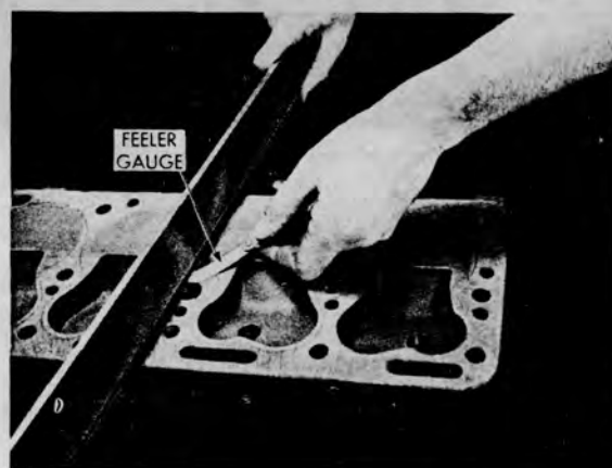
Figure 15 — Checking cylinder head flatness crosswise.
